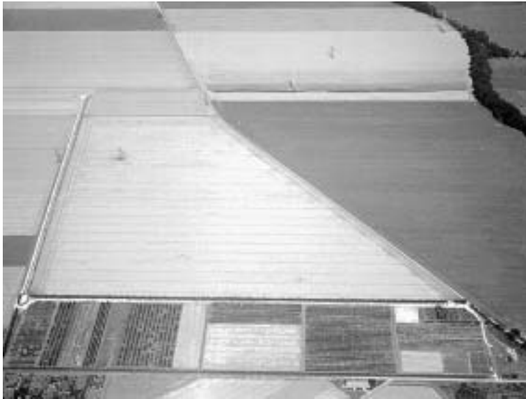
The aerial view clearly shows the general configuration of the Michelson-type interferometer. The vacuum tubes containing the 600-m interferometer arms are suspended inside a roofed trench by a wire pendulum from rollers running along a rail.
